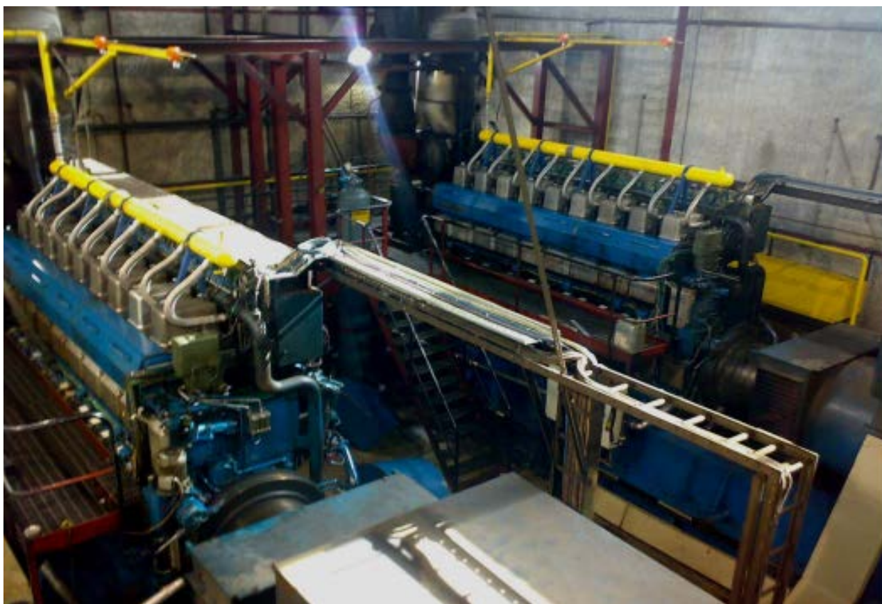
VTec Technology was used to convert two 4.0MW Diesel Engines to Natural Gas but can be used for H 2 at Estarreja Portugal.
